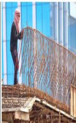
Hard at work: A labourer at work in Gurgaon, Haryana.
