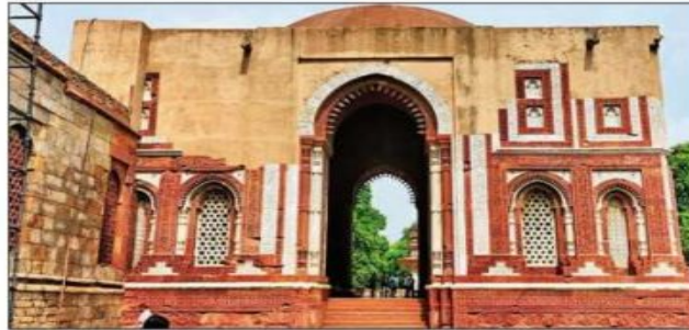
NIP & TUCK: In the first phase, handmade intricate carvings of red sandstones, which have eroded over time, will be replaced
