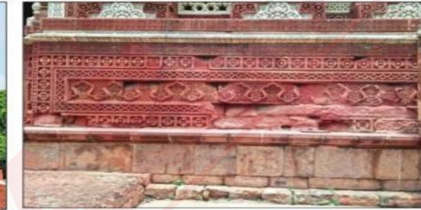
NIP & TUCK: In the first phase, handmade intricate carvings of red sandstones, which have eroded over time, will be replaced
